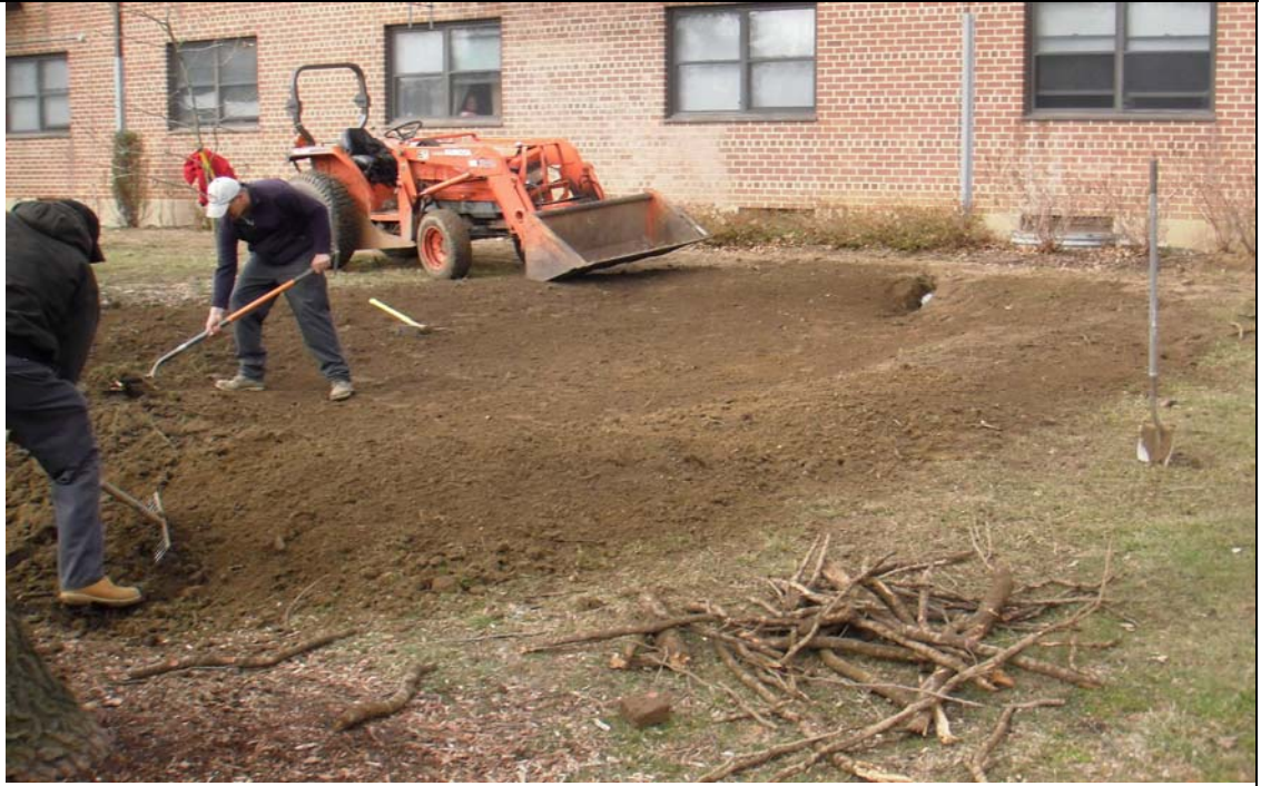
During Installati on
