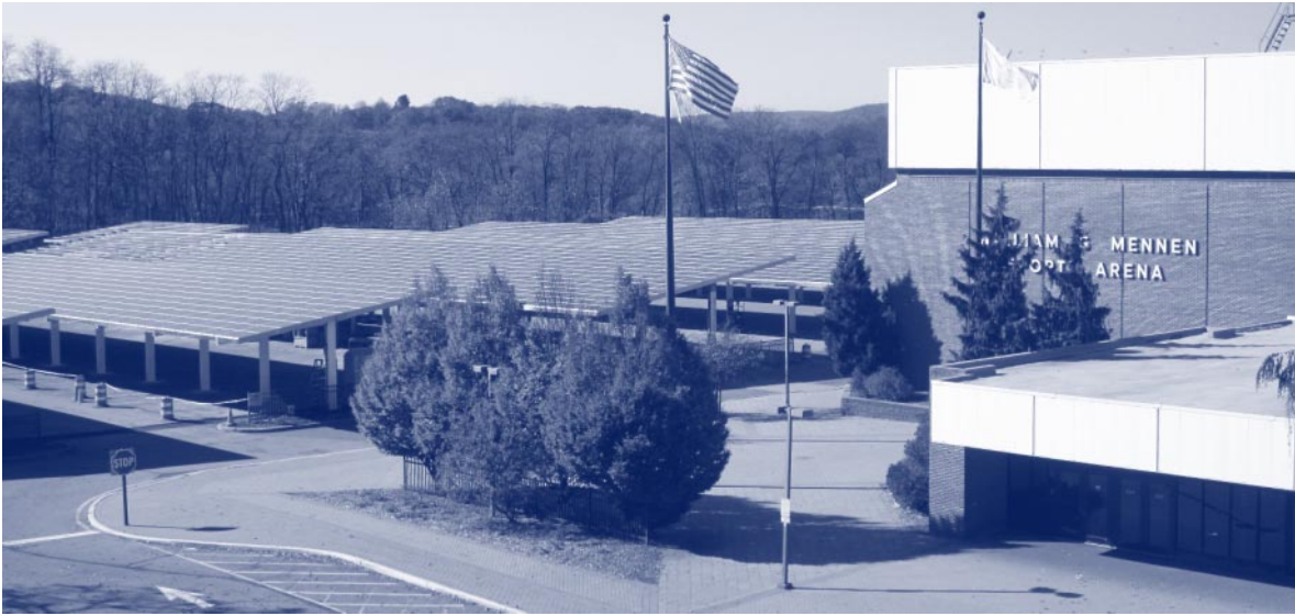
Solar panels on carport parking facility at Mennen Sports Arena in Morristown, NJ Morris County Park Commission
