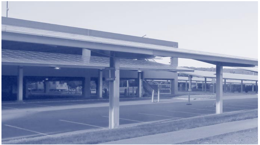
Solar panels on building and parking lot in Bridgewater, NJ Kerry Miller
