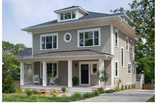
A Passive House Courtesy of David Peabody Passive House Institute & Alliance US
