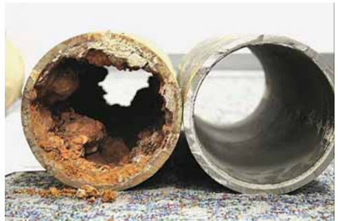
New Jersey's aging water infrastructure
