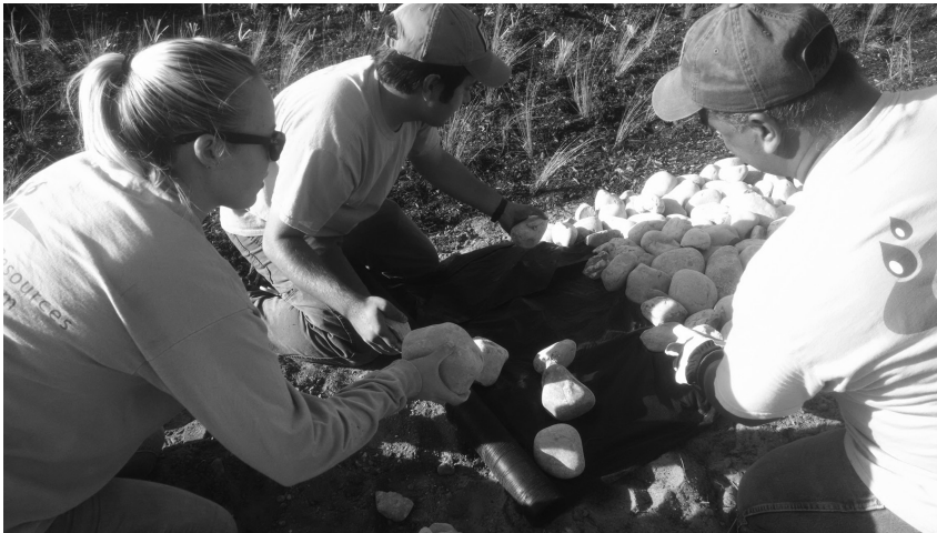
Pilesgrove constructing new rain garden
