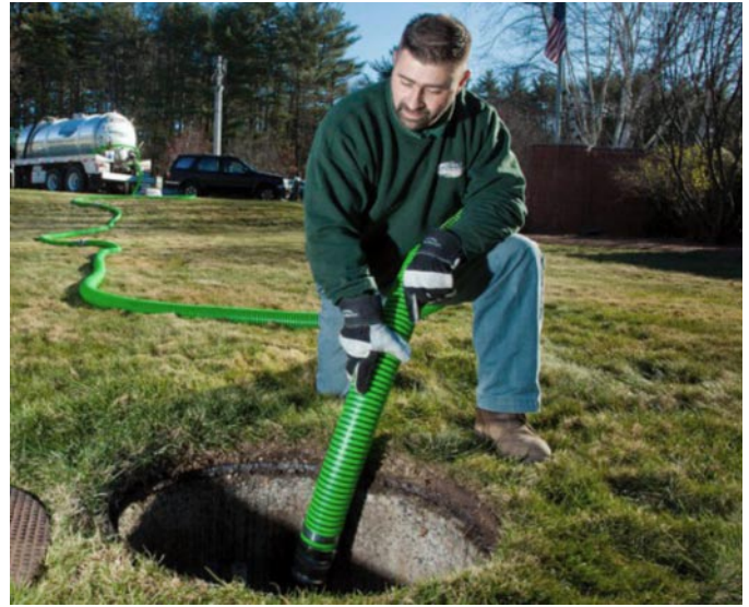
Septic Tank pumping Stock Photo
