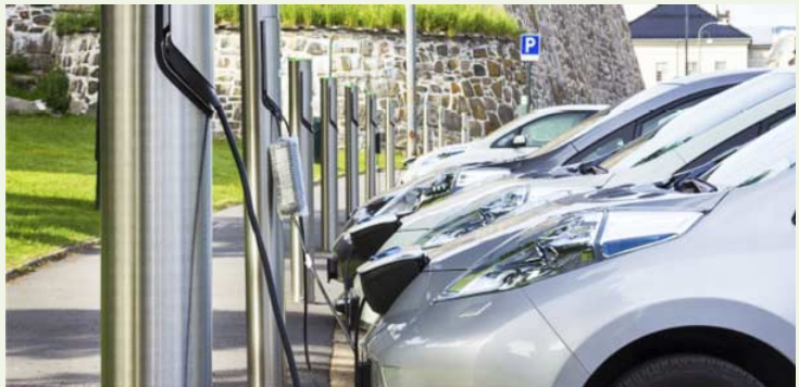
EV charging stations
