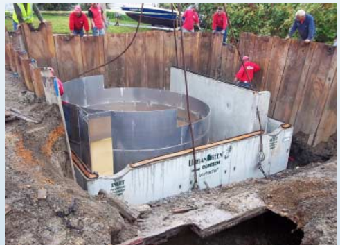
The Comstock Avenue helical swirl condenser, which removes sediment, litter, and particulate pollutants from Deal Lake
