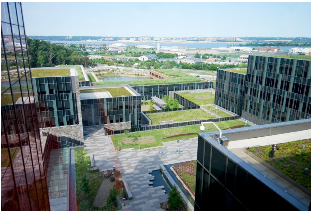
Photo 1: US Coast Guard HQ Washington DC layers on a green roof, of soil and plants can be as thin as just a few inches, or as thick as several feet depending on the structural capacity of the building and the types of plants that are used.
