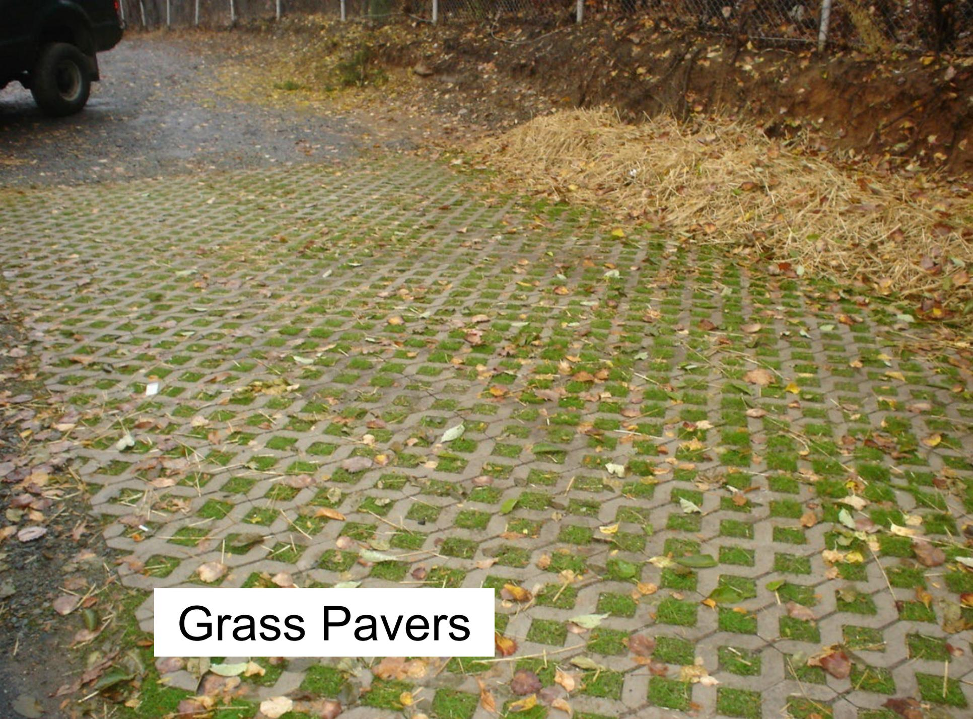
A photograph showing a driveway paved with interlocking concrete grass pavers. The pavers are arranged in a grid pattern, with green grass growing through the openings. The driveway is covered with fallen autumn leaves and some dry grass. In the background, there is a chain-link fence and a dark vehicle parked on the left side. The overall scene is outdoors during autumn.
