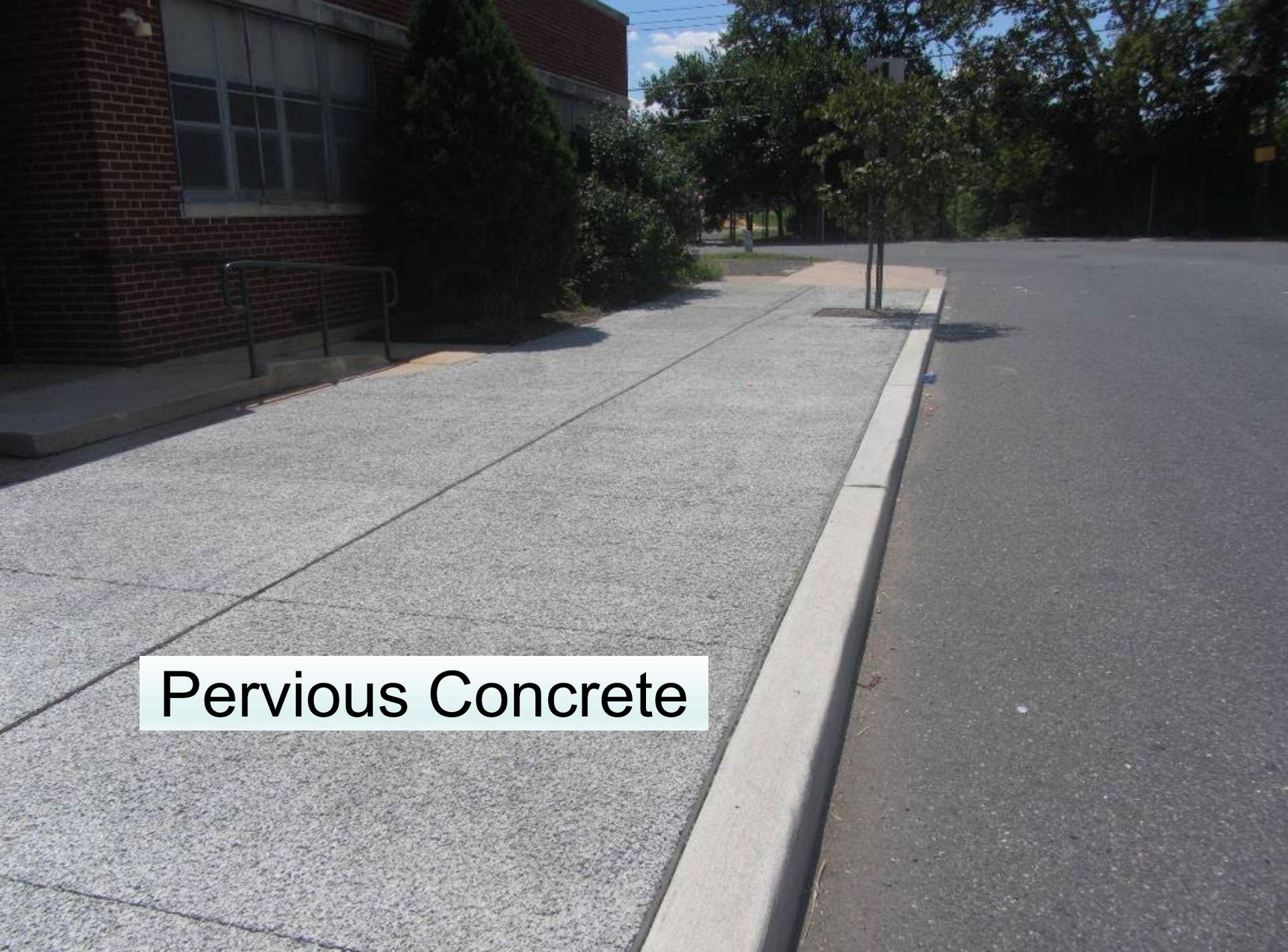
A photograph showing a sidewalk made of pervious concrete. The sidewalk is light gray and has a porous, aggregate-like texture. It runs alongside a brick building on the left, which has a metal railing. To the right of the sidewalk is a concrete curb and an asphalt road. The background shows trees and a clear sky.
