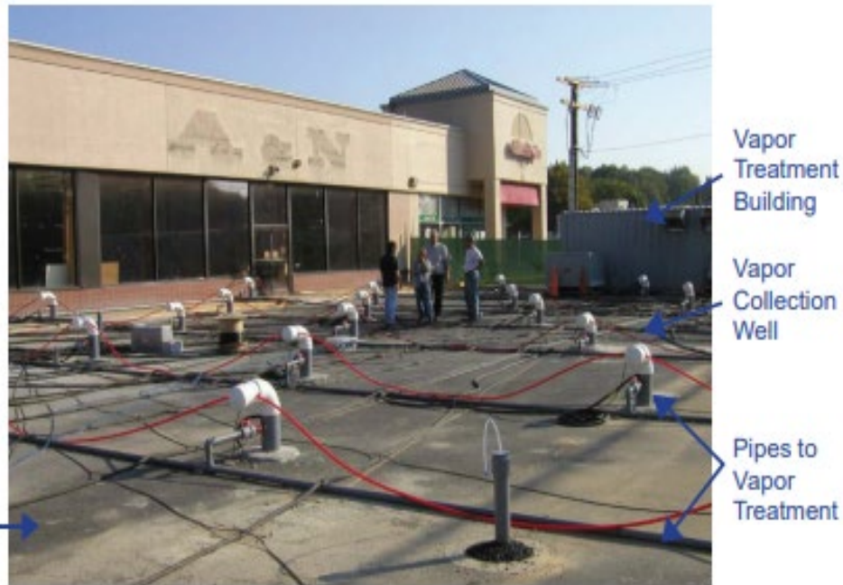
ERH system cleans up contaminated soil and groundwater.
