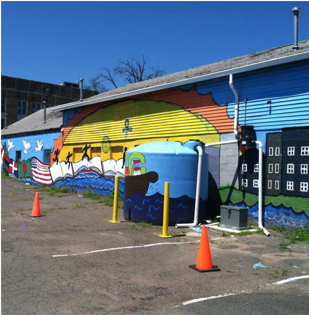
Cistern in Paterson, NJ
