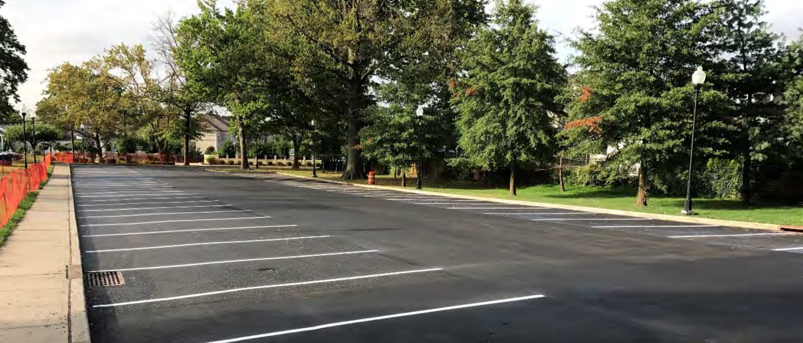
Porous asphalt parking lot at Washington Park, Perth Amboy, NJ
