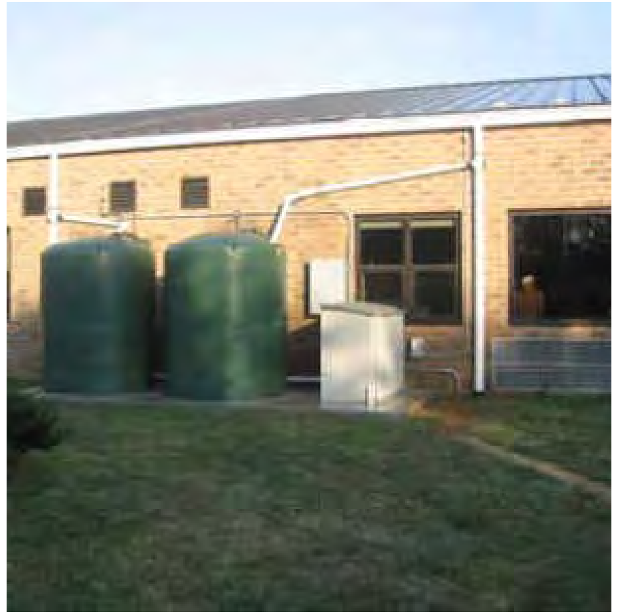
Cistern at a school in Greenwich, NJ
