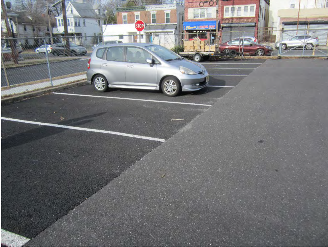
Porous asphalt parking lot on Westfield Ave, Camden, NJ
