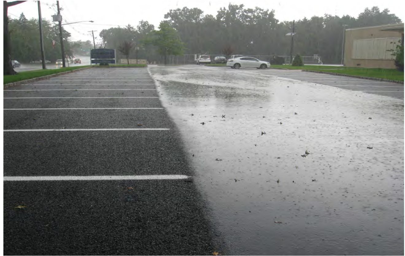
Porous asphalt parking lot at the Clark Municipal Building
