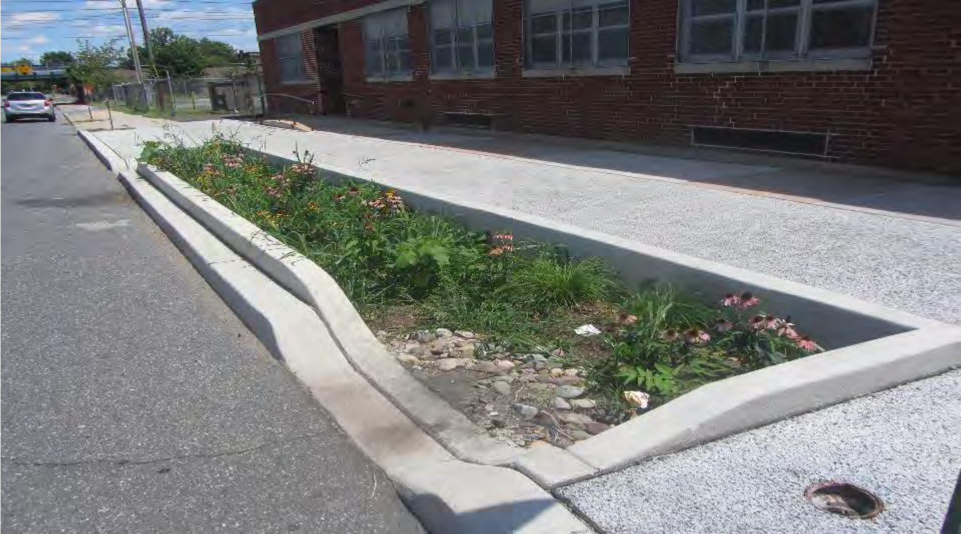
Stormwater Planter at the Brimm School Camden, NJ
