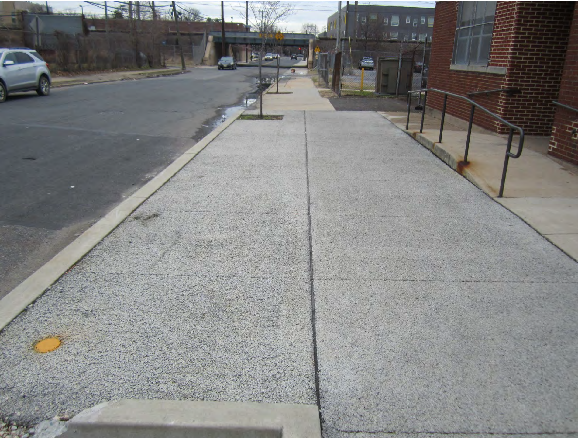
Pervious Concrete Dr. Charles E. Brimm Medical High School in Camden
