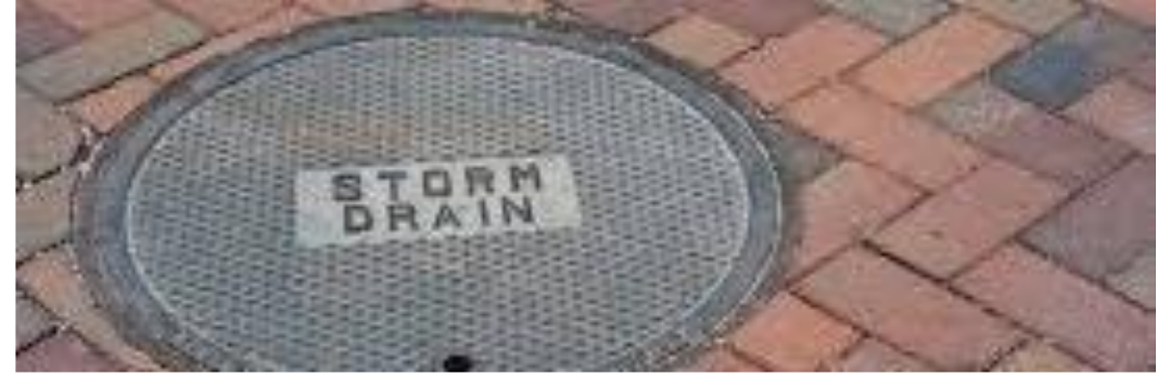
839 Storm Maintenance Holes
