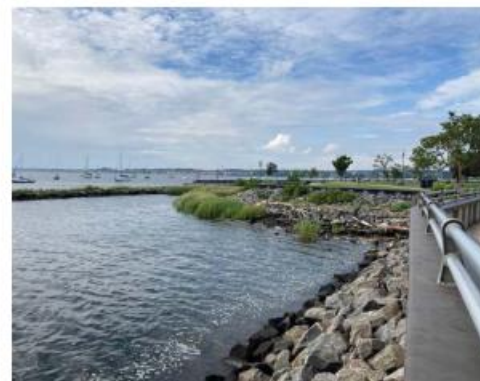
WATERFRONT BULKHEAD REPAIR Perth Amboy, NJ
