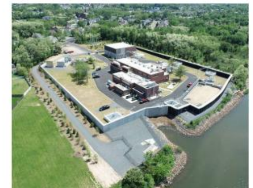
SAYREVILLE PUMP STATION Sayreville, NJ
