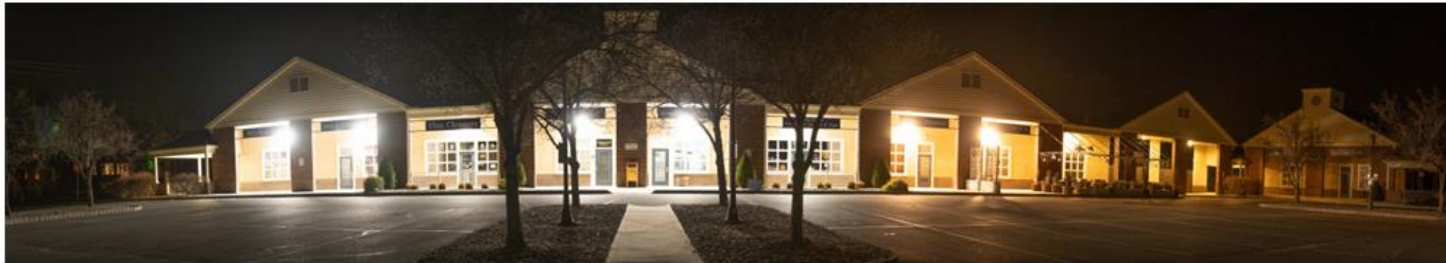
21 Mar 2025 10:30pm (parking lot lights off)
