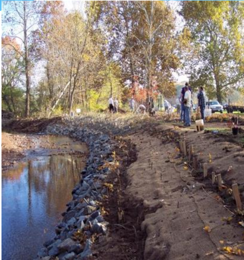
Walnut Brook, Mine Brook Park, Flemington, NJ Stream Restoration and Floodplain Reconnection
