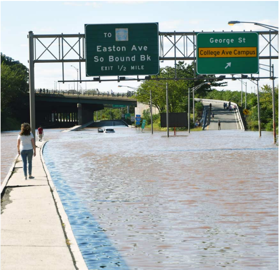
City of New Brunswick flooded after Hurricane Ida. IStock
