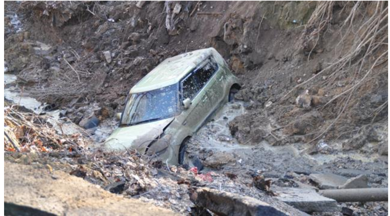
South Amboy (Gordon Street) 20-foot sinkhole caused by water main break, 2015
