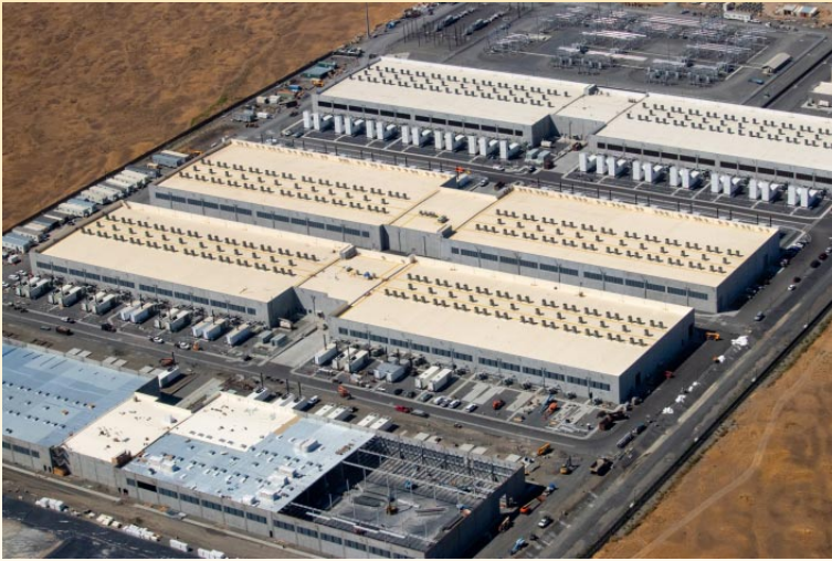
Amazon web services data center in Arizona
