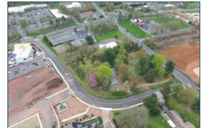
Route 206 & Route 518 - New Traffic Patt...
